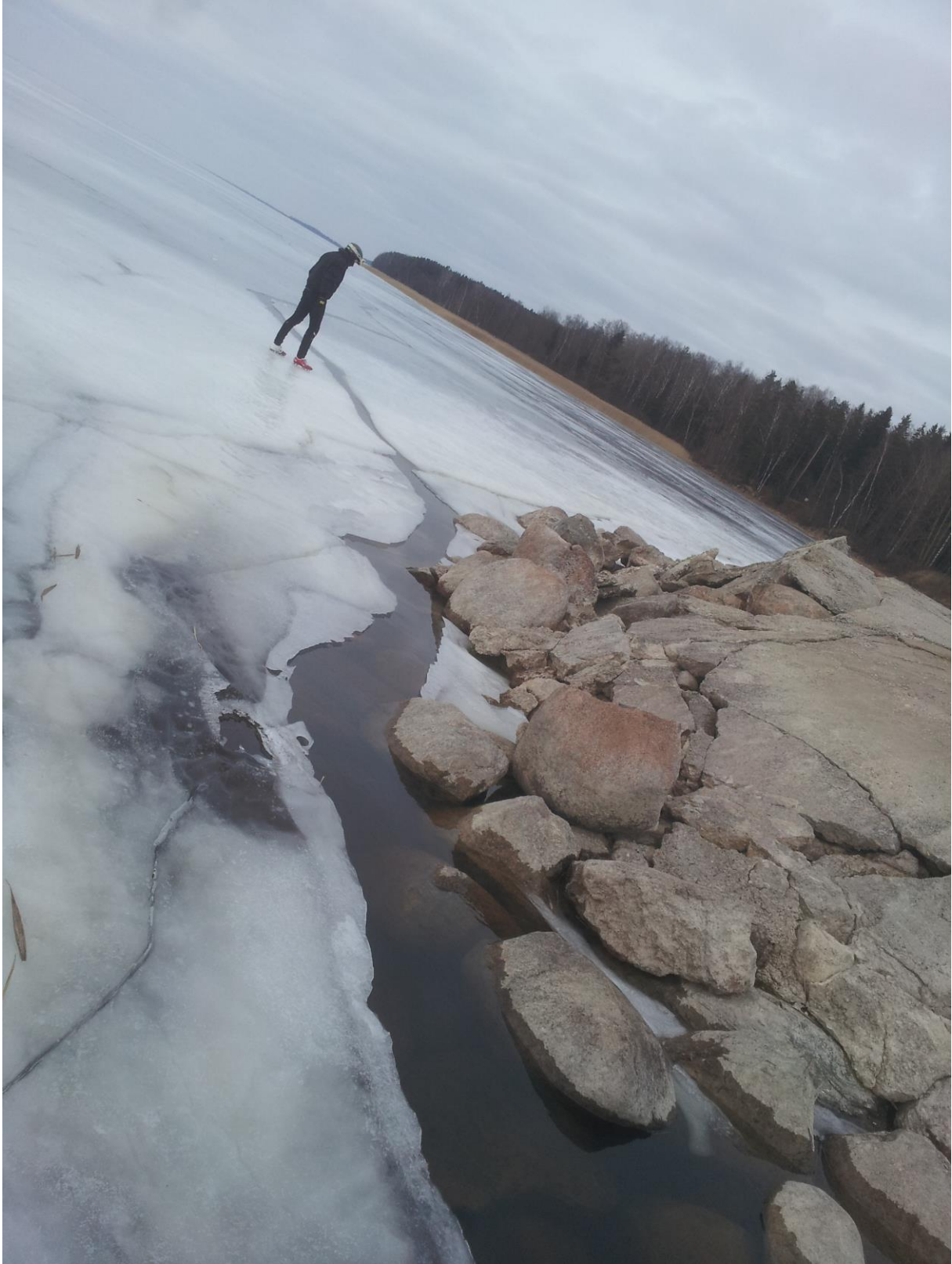
Pic 14. Jetty at Limnoliigia jaam (crack ends in about 100m)
